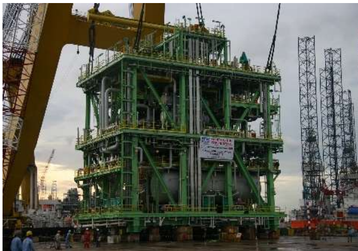
Oil Separation Module
